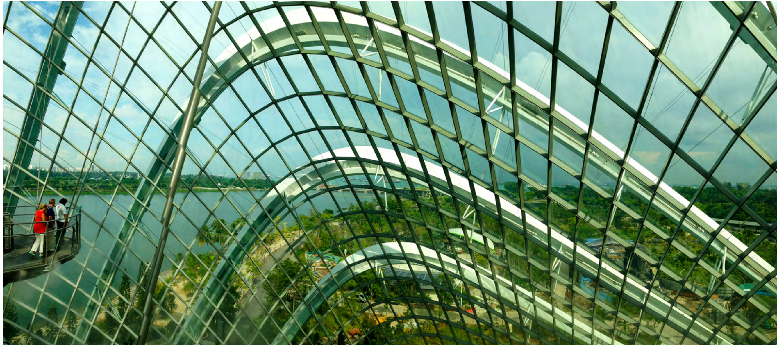
PHOTO BY SHINTA DJIWATAMPU
